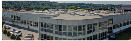
Plant I, Mindelheim, Germany
